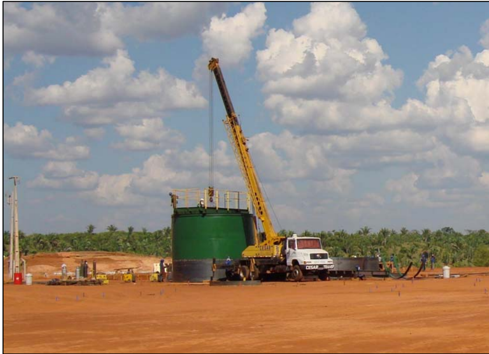
Figure 1: Andorinhas Mill site construction
